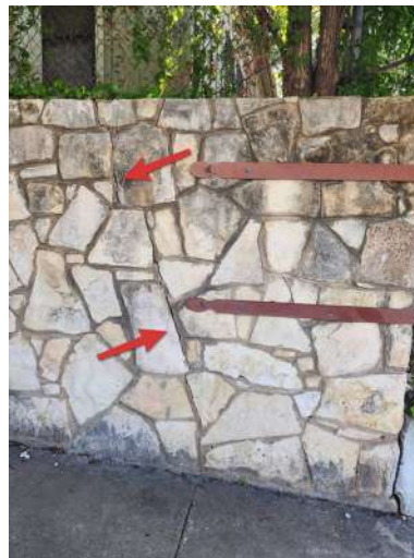
Front - retaining wall.
