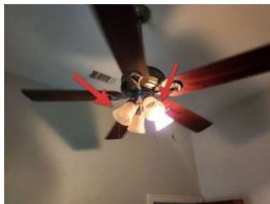
Bedroom - missing light bulbs.
