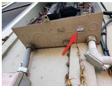
Missing knockout.
