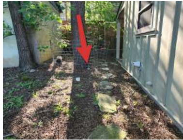
Left side - grading slopes toward the foundation.
