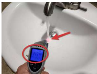
Hot water temperature - 143 F degrees.
