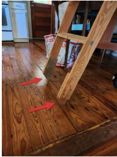
Attic access ladder.
