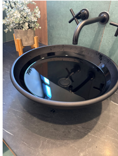
FLOOD TESTING CONDUCTED
