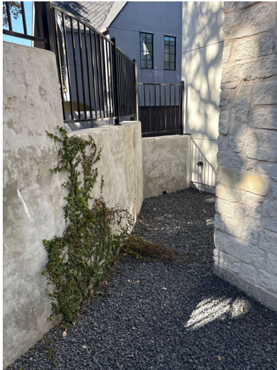
Retaining wall protecting rear of home
