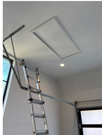
Garage attic not inspected -20ft A-frame ladder needed
