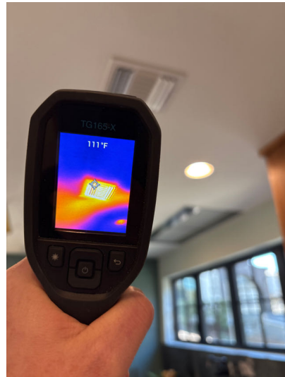
NORMAL THERMAL READINGS - DUCTS
