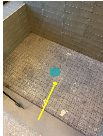
FLOOD TESTING CONDUCTED
