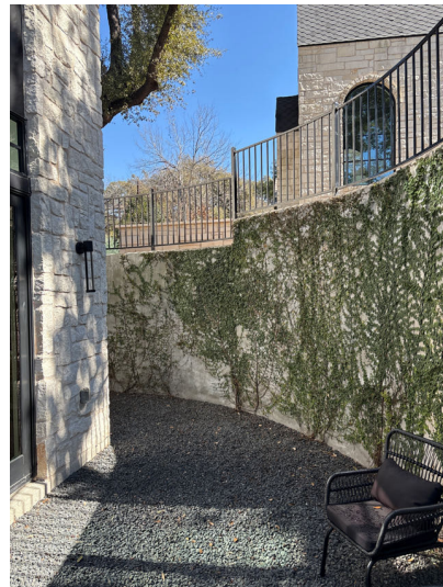
Retaining wall protecting rear of home
