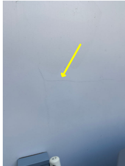
Stucco cracks
