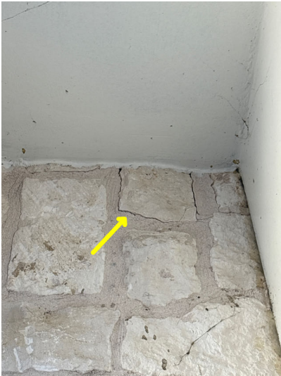
Mortar cracks/separation
