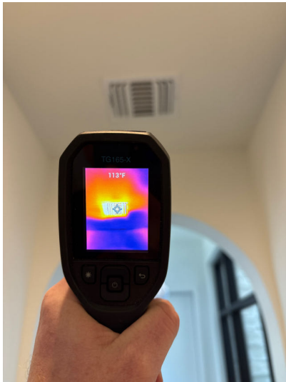
NORMAL THERMAL READINGS - DUCTS
