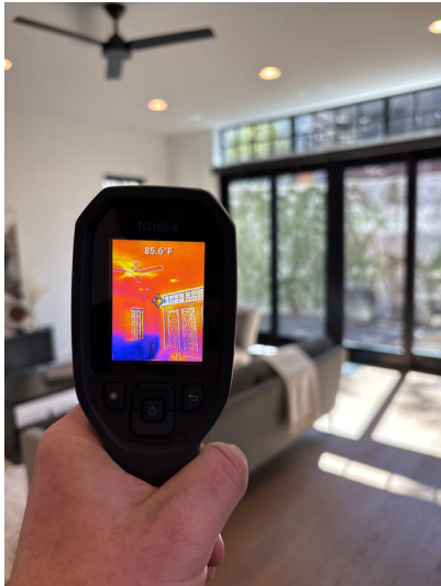
NORMAL THERMAL READINGS - INTERIOR
