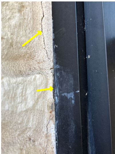
GAPS / CRACKS AT WINDOW SEALANT -first floor, multiple windows
