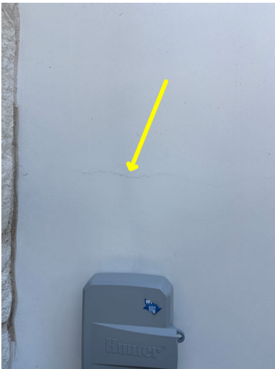
Stucco cracks
