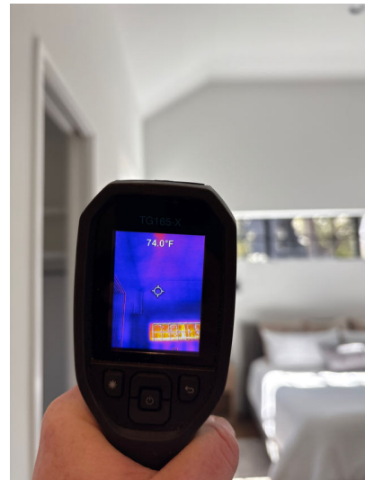
NORMAL THERMAL READINGS - INTERIOR
