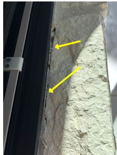
GAPS / CRACKS AT WINDOW SEALANT -primary bedroom
