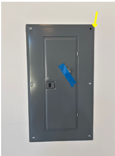
Missing fastener
