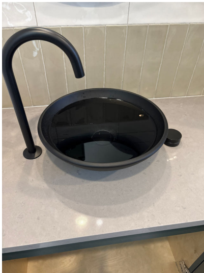
FLOOD TESTING CONDUCTED
