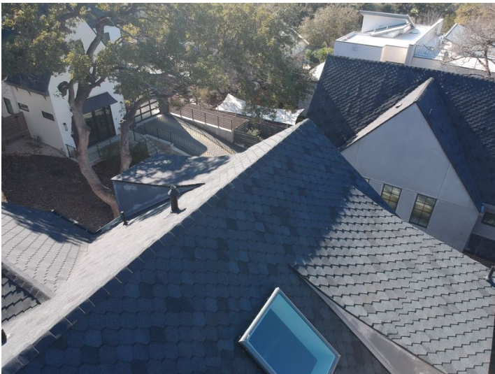
NO MAJOR ISSUES - SHINGLES
