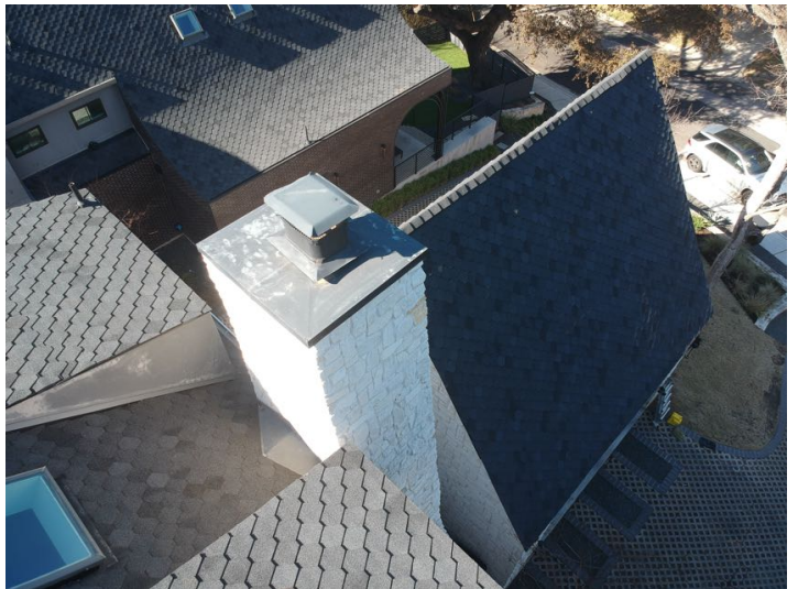
NO MAJOR ISSUES - ROOF
