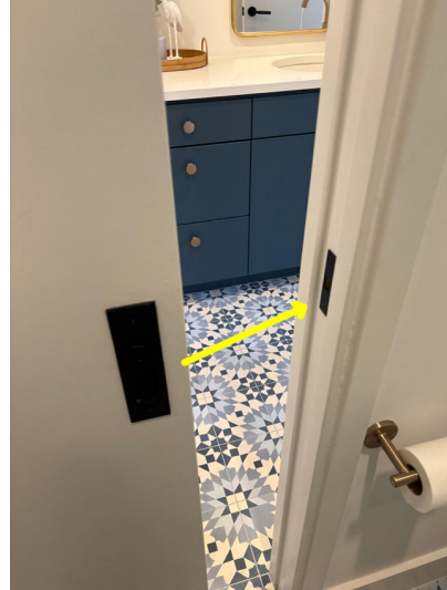
Lock and latch issue -Jack and Jill toilet
