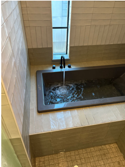
FLOOD TESTING CONDUCTED
