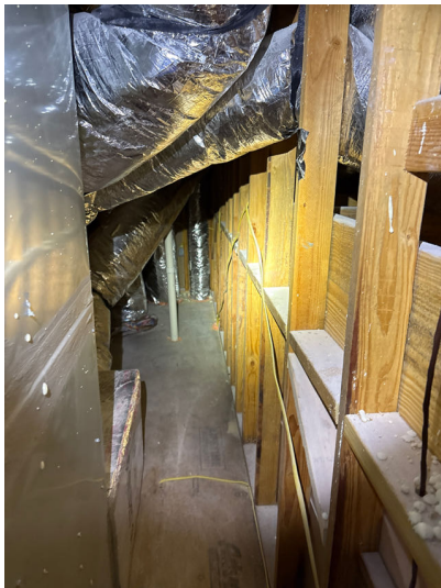
NO MAJOR ISSUES - FRAMING
