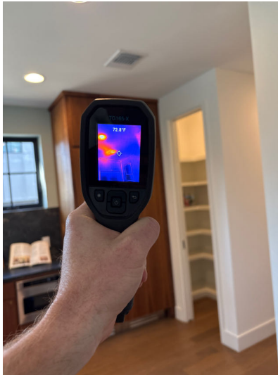
No moisture observed below shower/tub
