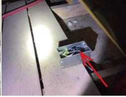
B. Outlets and Switches: The upper socket at the rear W corner master bedroom wall outlet did not function when tested. This outlet may be switched on at the light switch, however the switch did not appear to function for powering the outlet.
