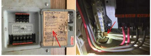
Type of Wiring: Aluminum Service Feed and Copper Branch Wiring
