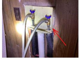
A. Exterior Plumbing Fixtures The front SE exterior hose bibs are not sealed and secured properly at the wall penetration, or insulated properly to prevent freezing.
